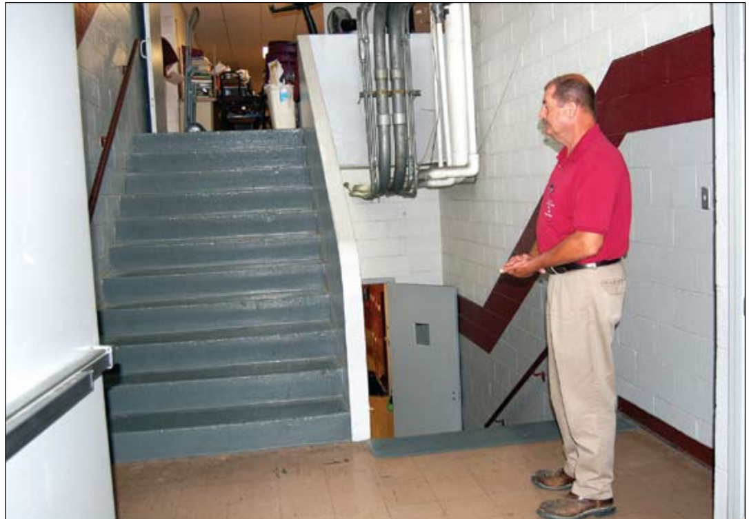
Metcalfe County Middle School has built onto several times so that now it has classrooms on five different levels, facilities director Herby Bunch said. The stairwell shows three different levels, as well as the piping installed to keep the building up to date with electrical needs.
