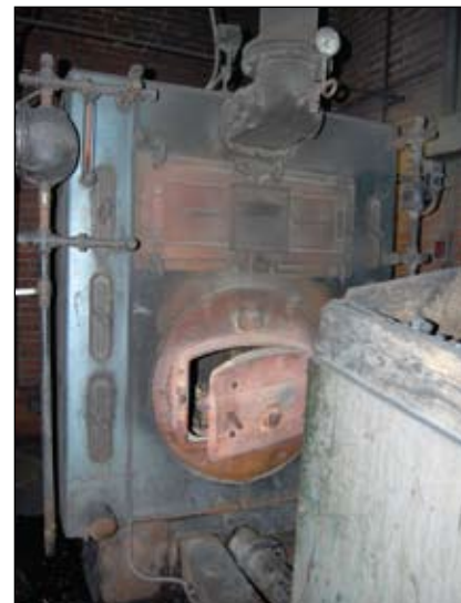
The 1925 coal-fired boiler at Ewing Elementary School in Fleming County battles to warm the entire school on cold days. Dust creates a problem for students with allergies and on very cold nights, the district has to have someone come in throughout the night to keep the fires burning and rooms as warm as possible. Read about Kentucky's category 5 facilities beginning on Page 12.
