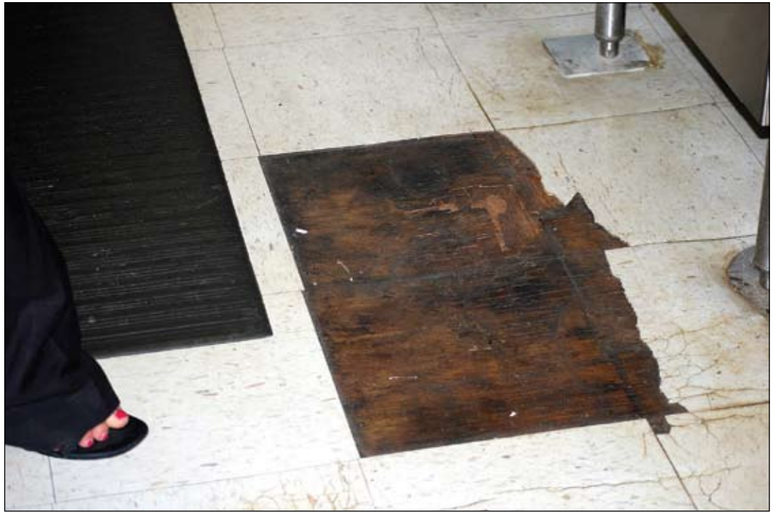
Moisture often gets under tiles in the kitchen at Fleming County’s Ewing Elementary School. Those tiles often break to expose the oiled wooden floors below.
